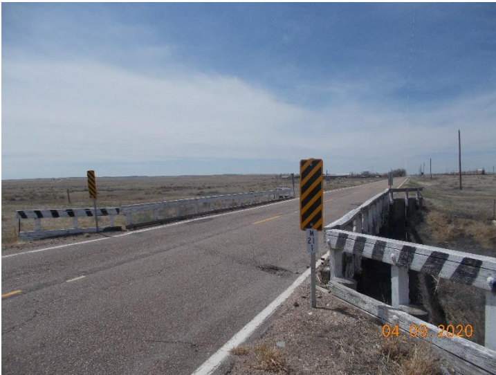
View of bridge M-21-I looking southwest.
