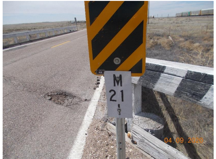
View of bridge M-21-I signage.
